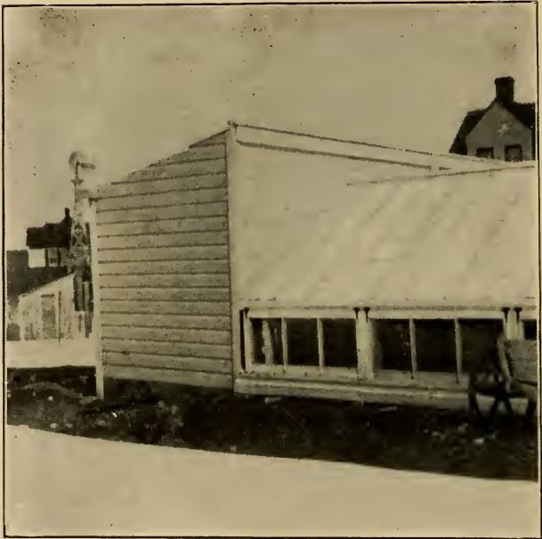
13.— Shed at north end of houses, showing method of construction. Shed has glass roof
